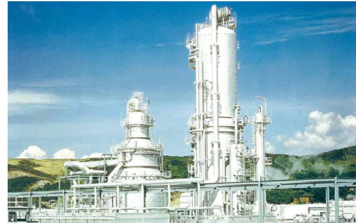
▲General view of oil refinery plant, including vacuum distillator tower on the left. 石油精製所、バキュームタワー(左)他に用いられた例
